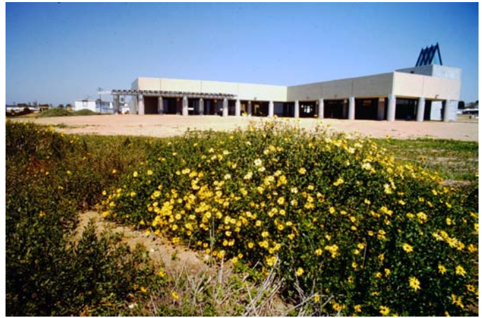
Fig. 18 -This view of the Visitor Center is almost finished in this view of early 1990.
