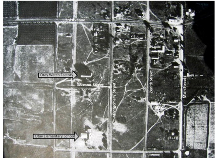
Figure 3 – Aerial Few of Otay 1928 (abandoned Otay Watch factory building in center of photo).
