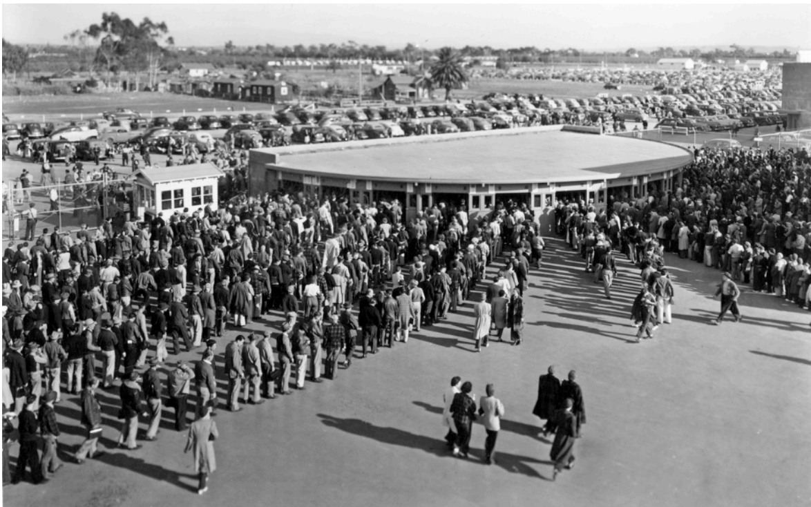
Rohr employees lined up each week at the clockhouse next to the H Street gate and guardhouse to receive paychecks until the clockhouse was demolished in 1959. In the middle of the parking lot beyond the clockhouse is the home of John Becerra who refused to sell his quarter acre and instead charged $1.50 per week for parking (earning enough to send his kids to college).
