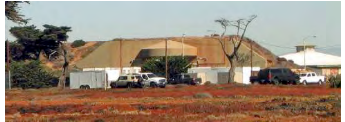
The bunkers at Fort Emory were built in 1942 on the former site of Coronado Heights to house coastal defense guns manned by the 19th Coast Artillery. The base was transferred to the Navy in 1950 and became part of the Naval Radio Receiving Station that had been established in 1920.
