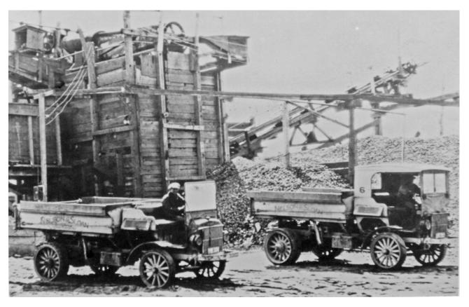
Above, the Nelson & Sloan plant in the Otay Valley in the 1920s crushed rock brought to the plant by railroad dinkies and transported from the plant in dump trucks. Below, the great conveyor belts built in the 1960s finally stopped in 2003 when stone from Rock Mountain was no longer processed at the 60-acre Nelson & Sloan plant.
